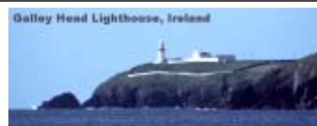
Galley Head Lighthouse. Galley Head Lighthouse is beautifully situated on the tip of a peninsula on the rugged southwestern coast of Ireland. The lighthouse was first established in 1878 and is 21 meters high. The light is 53 meters above mean high water and has a range of 23 nautical miles. The lighthouse became unwatched on 31st January 1997.
